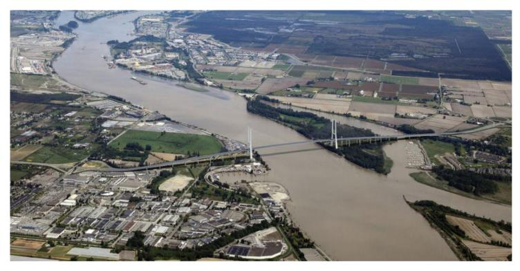
Three spans cable stayed bridge for the replacement of the existent tunnel. Main span with 634m length
